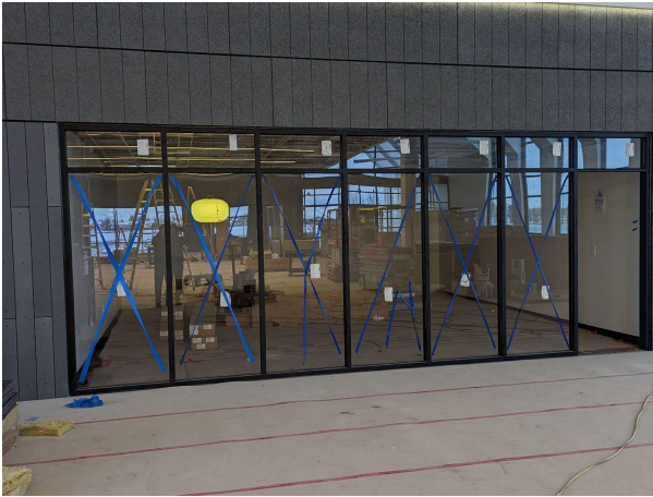
Windows installation in the large meeting room and the program room
